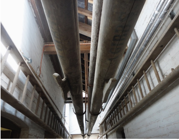
Fig. 10 Masts from clippers owned by the Gibbs and Sons merchant house, Tynesfield, UK (Purbrick 2013).
